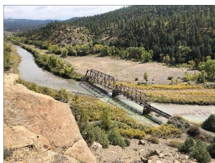
Double Truss Bridge
